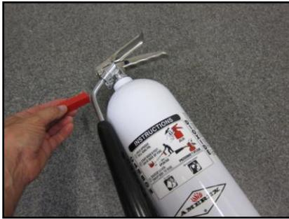
Figure 6. Testing extinguisher with small magnet
